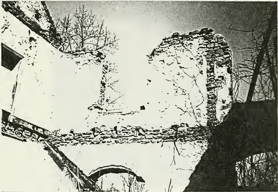
Figure 32: Interior view of window along east elevation
